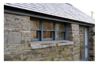
If it is necessary to close an original opening, it will be appropriate to use a recessed panel to indicate where the original opening was located.
