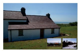
Where lime mortar has originally been used as part of the building construction any repointing or repair should use this material rather than cement.
