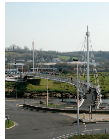
Pont King Morgan Carmarthen: a modern, visually pleasing addition to the townscape and landscape providing pedestrian and cycle links from the railway station to the town centre.
