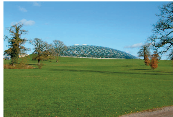
National Botanic Gardens: The impressive glass dome is a major piece of modern architecture which provides a contrasting yet iconic addition to the area's sense of place.
