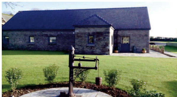
Modern restoration of a farmhouse that has re-interpreted traditional styles.
