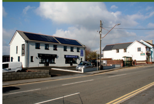
Mixed use frontage development with residential above the shops.
