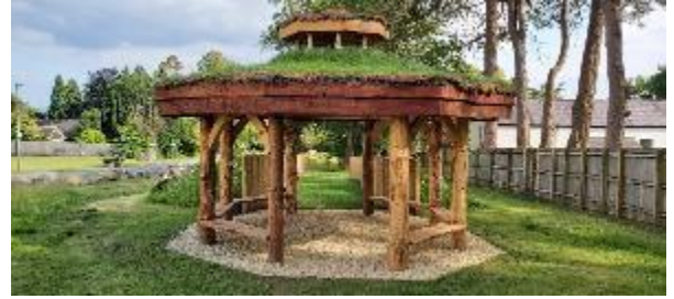
Shelter with a green roof built by the Biophilic Wales project
