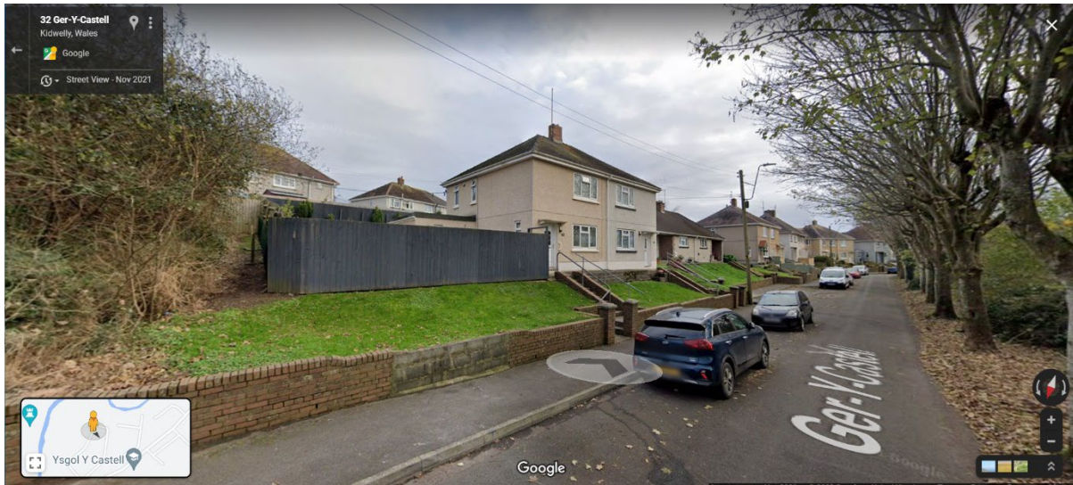
Figure 38 – Photo of 32 Ger Y Castell that had internal flooding from the rear.
