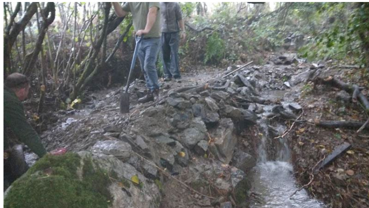
Figure 24 – Photo of Kidwelly residents unblocking the Cae Ffynnon watercourse north of Cae Ffynnon. In the picture, the water is flowing down the footpath, the watercourse is where the men are standing.
