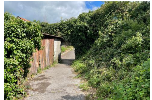
Remains of masonry wall to the north of Castle Farm
