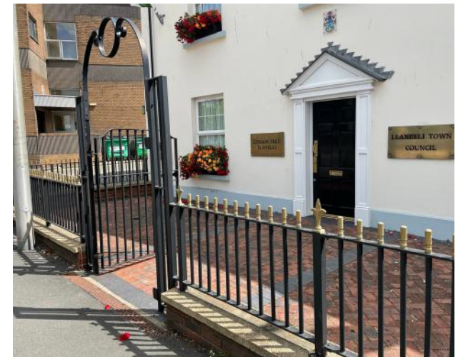
Metal railings at the Old Vicarage
