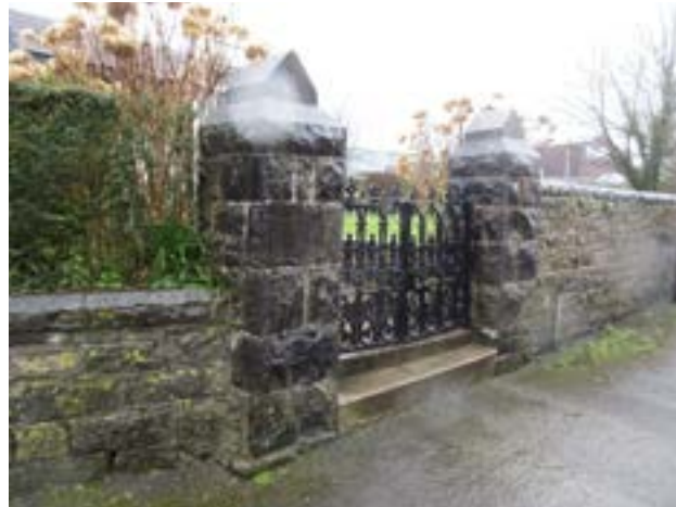
Coursed rubble wall, piers and gate to former 'Capel Penuel'
