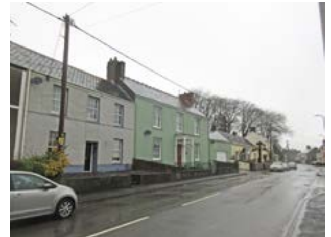
Shallow forecourts along Bridge Street
