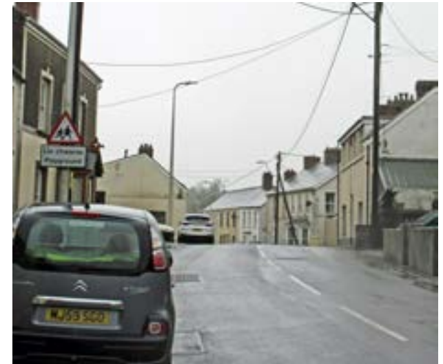
Steel lamp posts and overhead power lines
