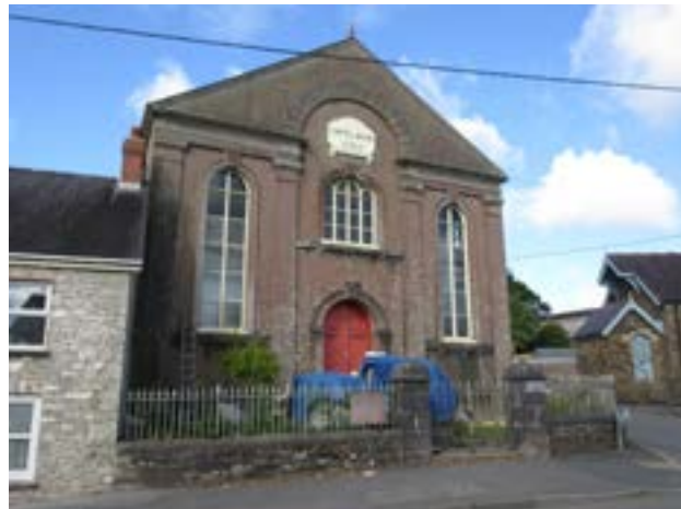
Snecked stone wall, piers, gate and railings to Capel Mair
