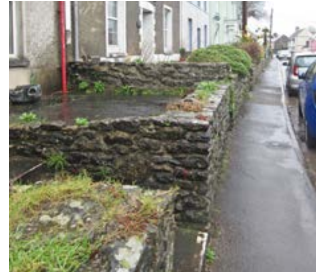
Rubble stone boundary walls on Bridge Street
