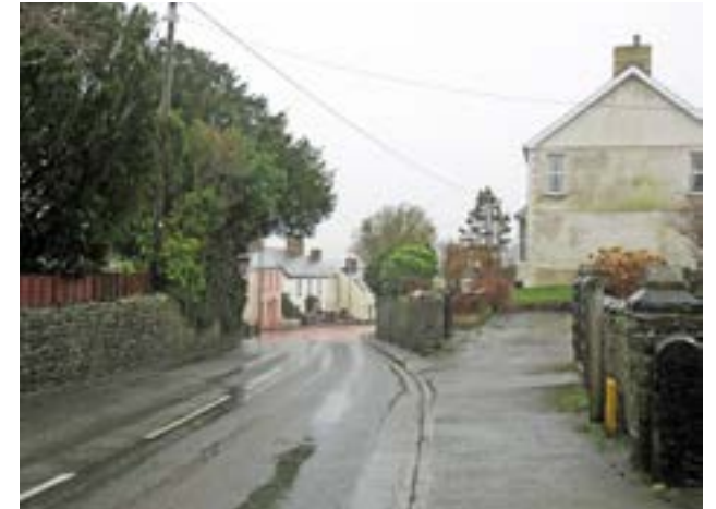
Rubble stone retaining wall at top of High Street
