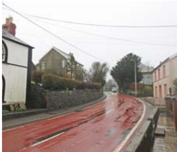
Coloured tarmac at top of High St, concrete kerbs, intermittent pavement
