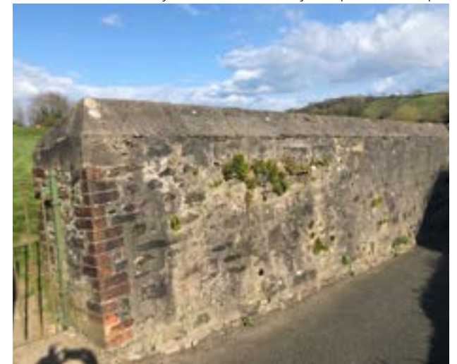
Boundary wall to the allotment gardens
