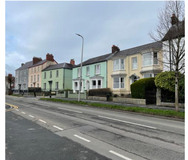
Metal railings to Picton Terrace
