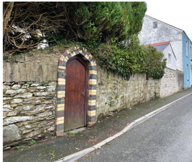
Rear gate and boundary wall on Picton Place
