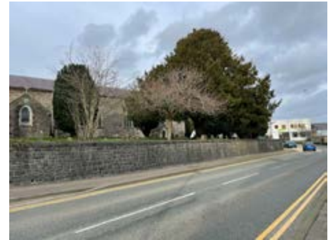
Stone boundary wall to St Peter's Church
