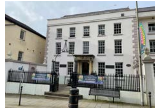
Metal railings to Carmarthen library
