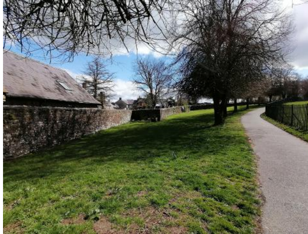
Rubble stone wall and open metal fencing
