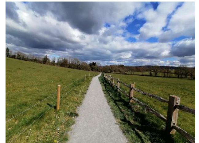
Timber and post and wire fences
