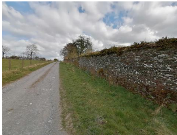
Rubble stone wall
