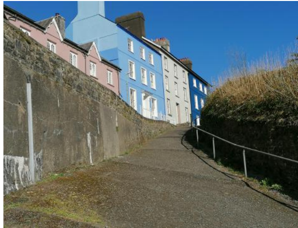
Chipped tarmac to Bank Buildings
