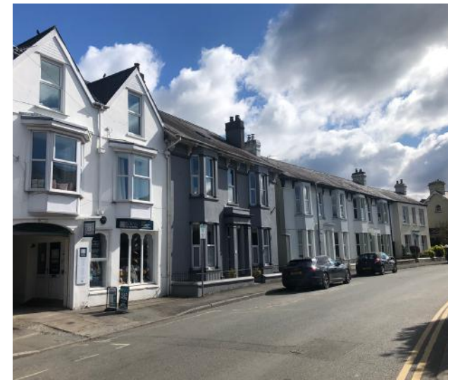
Crescent Road looking east
