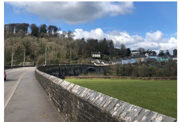
Llandeilo Bridge looking towards Bridge Street
