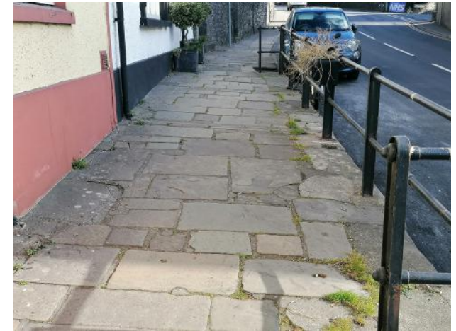
Stone slabs to Bridge Street
