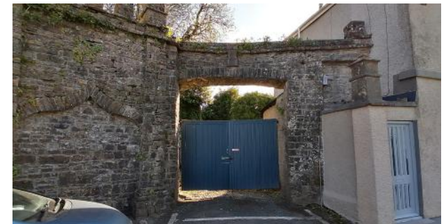
Crenelated masonry wall to Abbey Terrace
