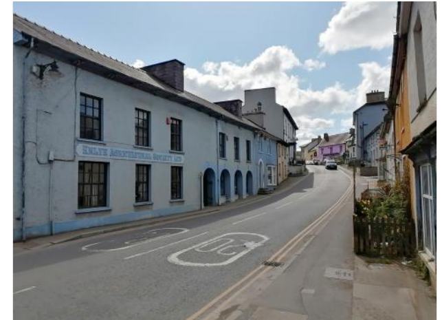
View north along Bridge Street
