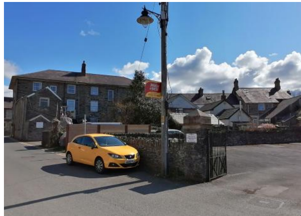
Boundary wall and gates to Bethel Presbyterian Chapel
