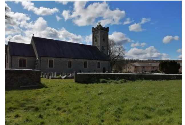
Boundary wall to Holy Trinity Church
