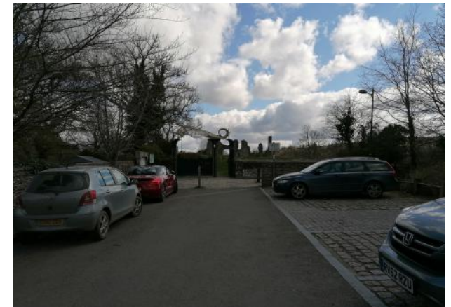
Stone setts, slabs and tarmac at Castle Street
